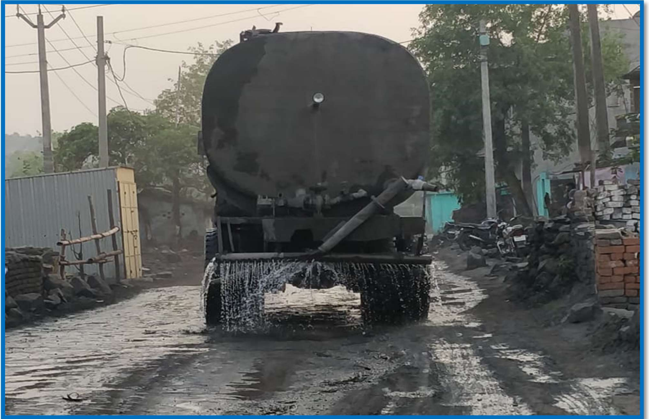
Picture 4 (I) – Water Sprinkling on Transportation Road
