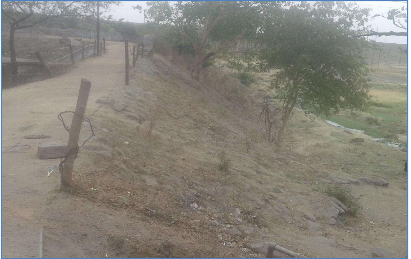
Picture 5 - Stone Pitching/embankment at Kari Jore
